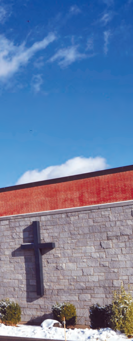
◀ The former St. Mary School in Newington now houses a Catholic Charities program for people with disabilities.
